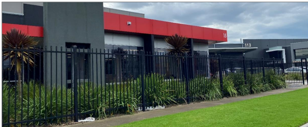
Figure 61: Vanguard fencing combined with low planting provides a high quality and permeable interface to the street.
