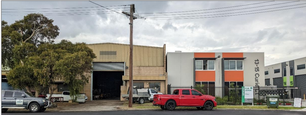
Figure 55: Example of mixed built form styles at Seaford and Seaford North.
