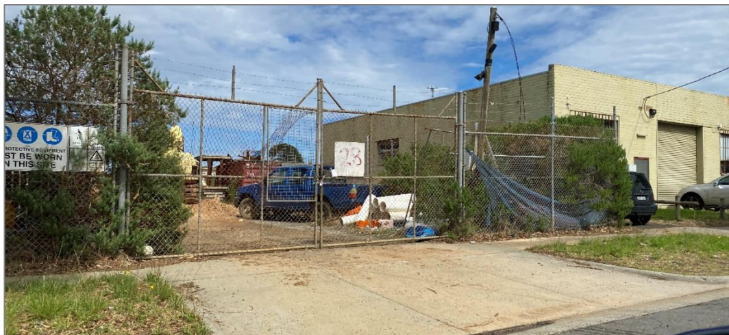
Figure 62: While permeable, chain mesh fencing presents poorly to the street.
