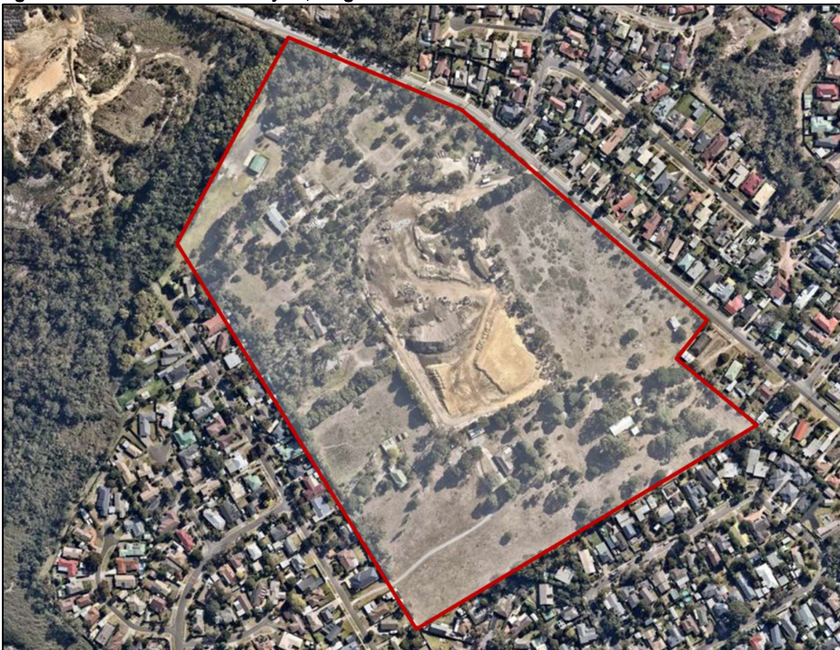
Figure 14: 18 Ha site on 75 Quarry Rd, Langwarrin
