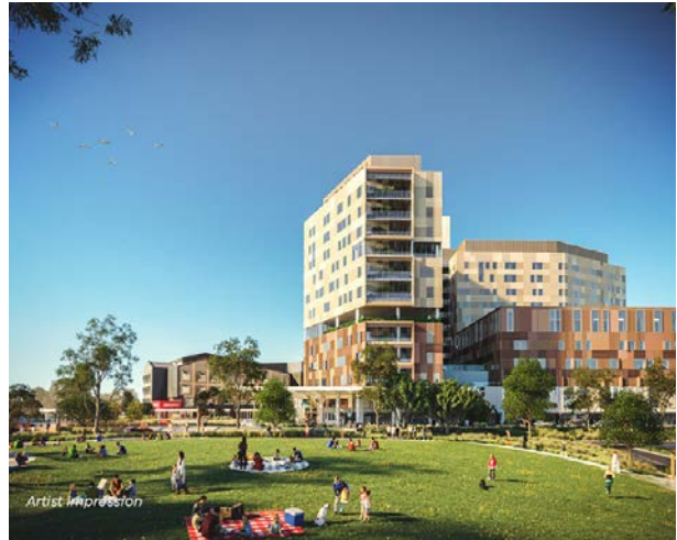
Frankston Hospital Redevelopment - Victorian Health Building Authority.
