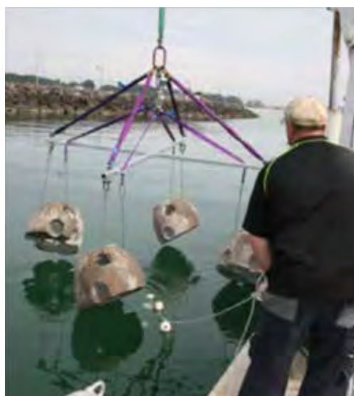
Installation of similar reef modules. The State of Victoria.
