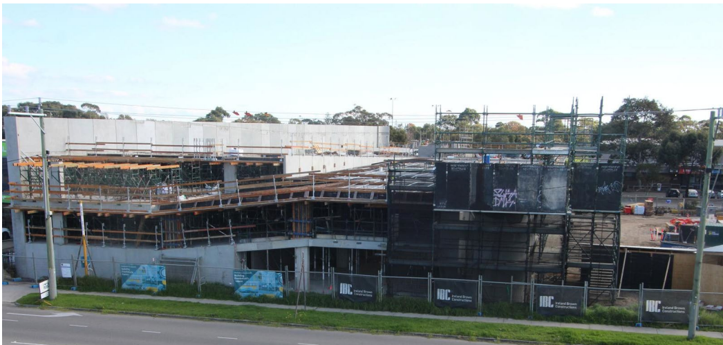
Construction as at 6 May 2024.
