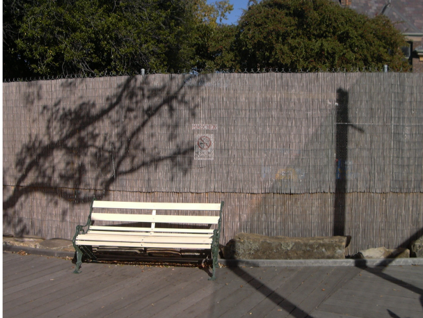
Fine 'matchstick' on cyclone wire: note its semi-transparency, ability to filter winds, and 'shadow wall' qualities which contribute vitality
