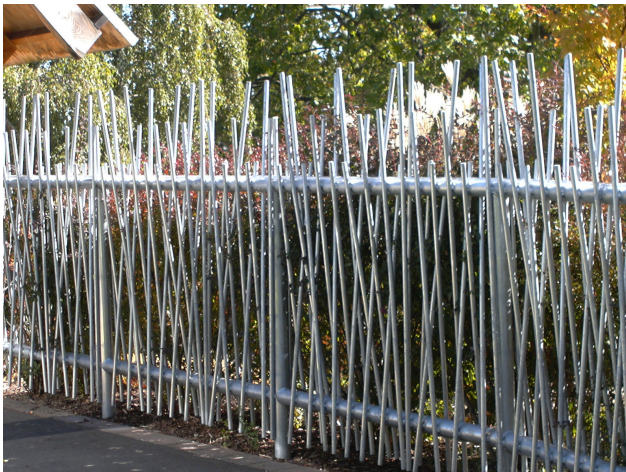
A contemporary interpretation of the tea-tree fence, in steel construction
