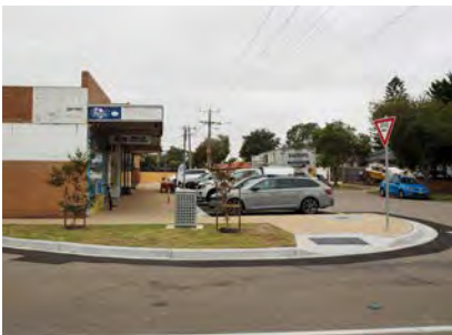
Recently completed outstand with additional tree planting
