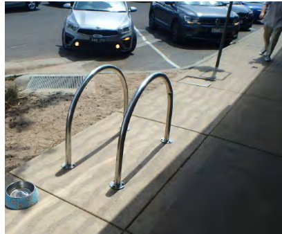
Feature paving and bicycle facilities
