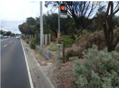
Poor connections to bus stop
