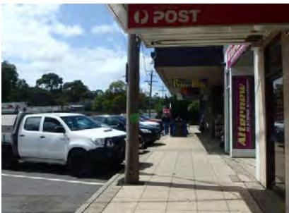
Regular openings, windows and entries
