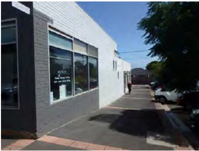
Lack of activation along Omaroo Road
