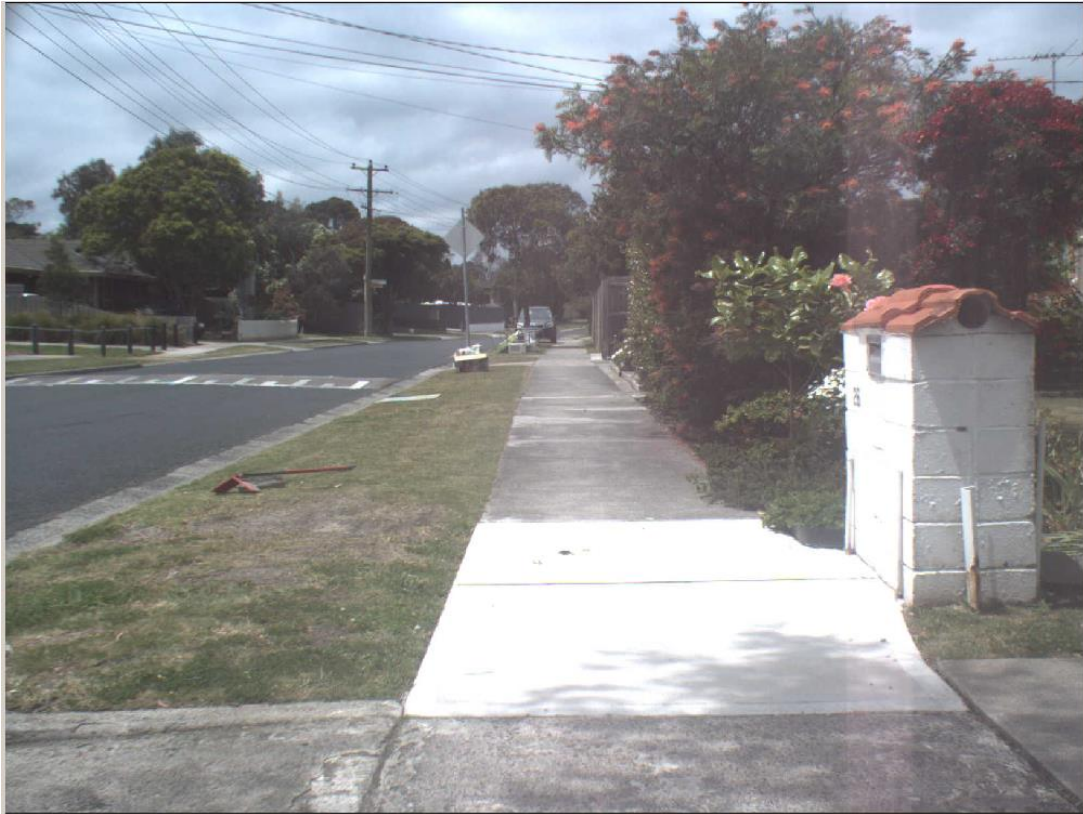
Footpath 22070,1,1 – Jacana Avenue, Frankston – Segment is 50 years old, assessed as condition 2
