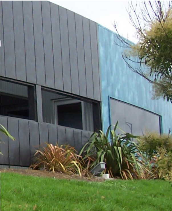
Textured concrete combined with windows and openings is utilised in this example to provide for articulation of the facade
