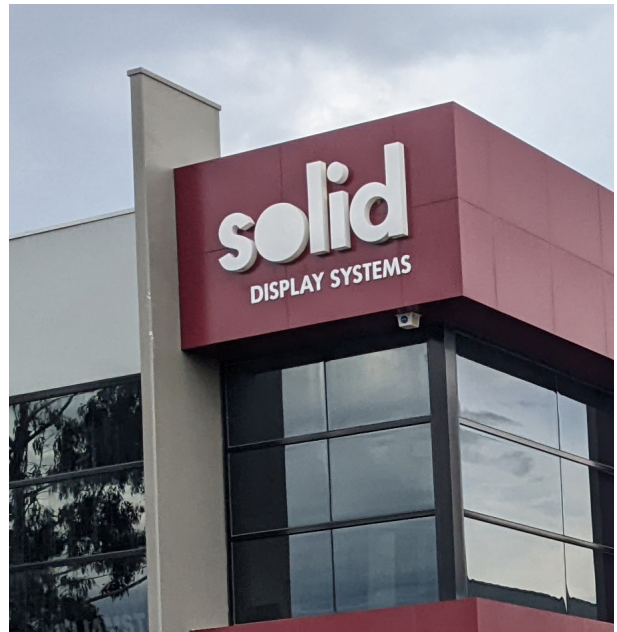
An example of directional signage that integrated into the building design.
