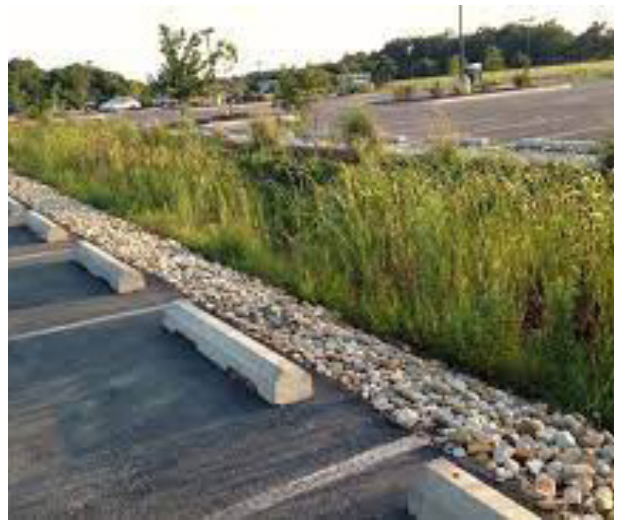
Locating a naturally vegetated swale within a car park increases visual amenity whilst providing passive infiltration.
