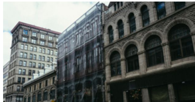
Heritage Building Restoration in Montreal
