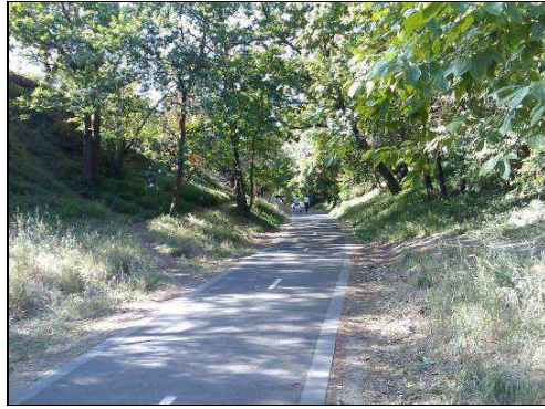
Figure 8.5 Bitumen with concrete edges
