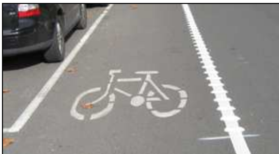
Figure 8.1 Profiled edge lining as applied to a bicycle lane on Rathdowne Street in the City of Melbourne Source: Bicycle Victoria
