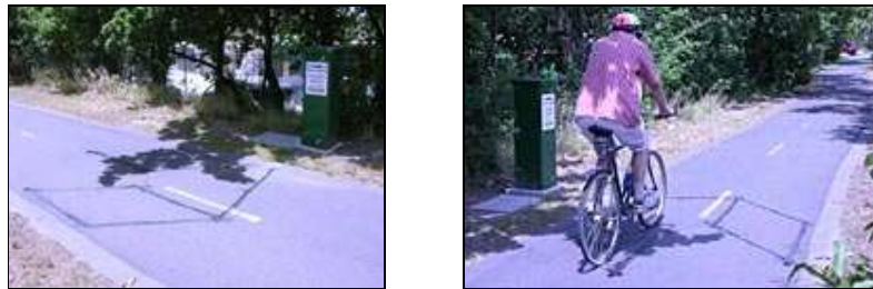
Figure 7.2 Bicycle detector loops on an off-road path in Melbourne
