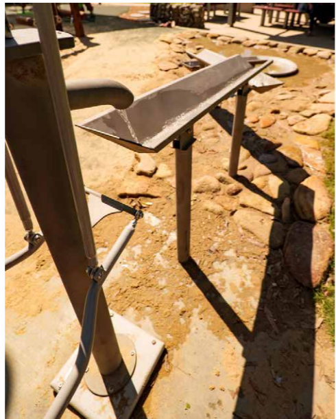
Water play hand pump connecting to stainless steel troughs with final outlet directed to planted swale
