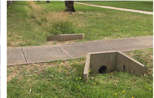
5. Grass swale directing storm-water south along western boundary
