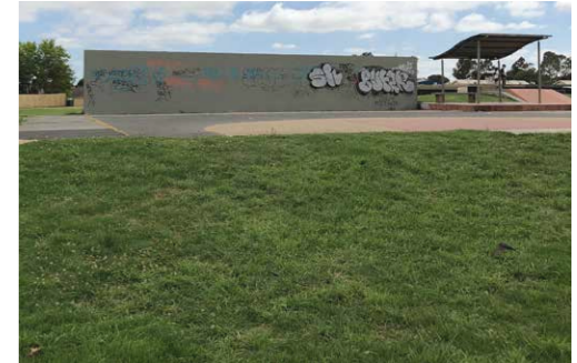
7. Large rebound wall part of active play / half court area to be removed (future)
