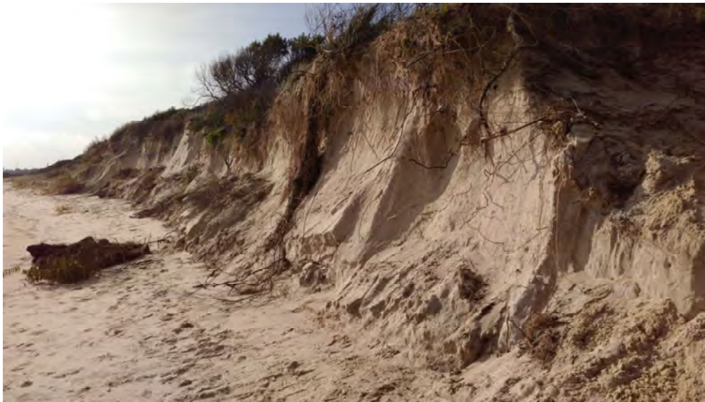
Figure 6-2 Example of coastal erosion of beach and dunes into the vegetation reserve, Seaford foreshore
