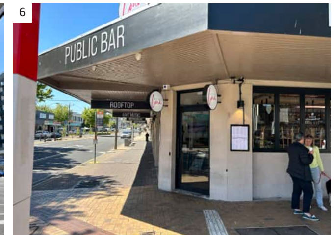
6 Nepean Hwy CBD canopies with no lighting
