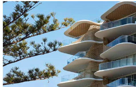
Example of coastal design aesthetic and materials, with light and natural materials with interesting forms and consideration of specific local environmental issues.
