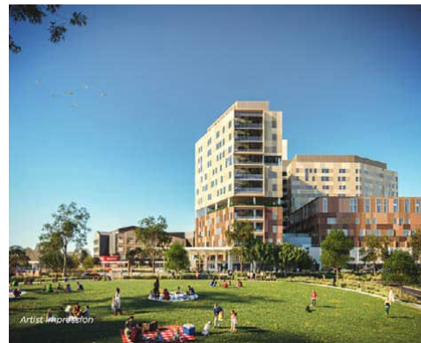
Frankston Hospital Redevelopment - Victorian Health Building Authority.
