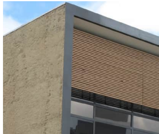
An example of simple detailing and form
