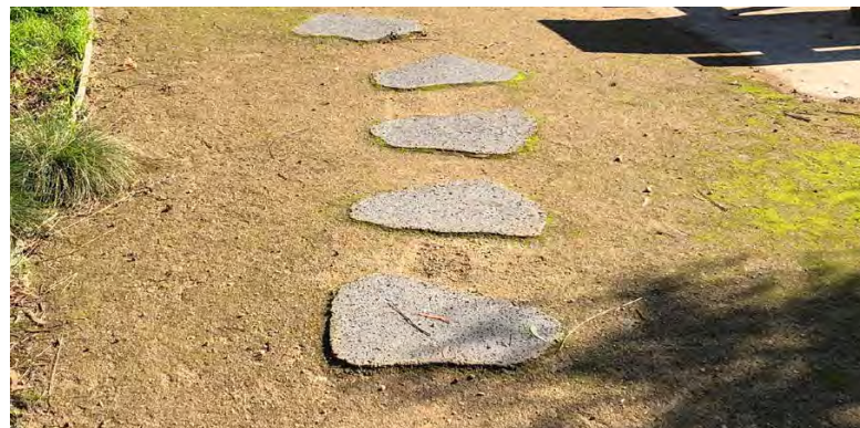
Stone stepper in granitic gravel to be replaced with accessible sealed pathway
