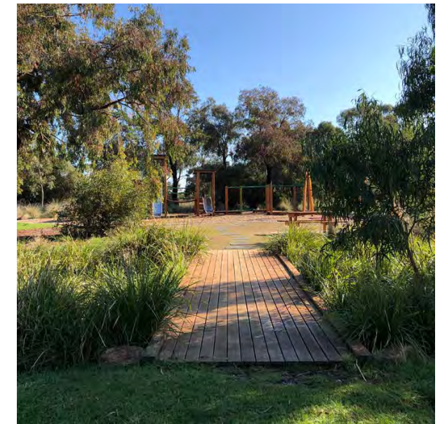
Existing timber bridge over swale does not connect to accessible sealed pathway
