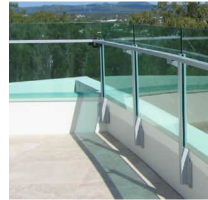
BA 01 - GLASS BALUSTRADE WITH BACK STRUCTURE.
