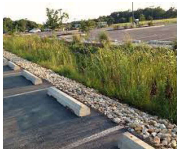
Locating a naturally vegetated swale within a car park increases visual amenity whilst providing passive infiltration.
