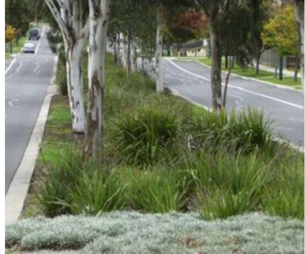
Vegetated median incorporated into the road reserve will passively treat storm-water run-off.
