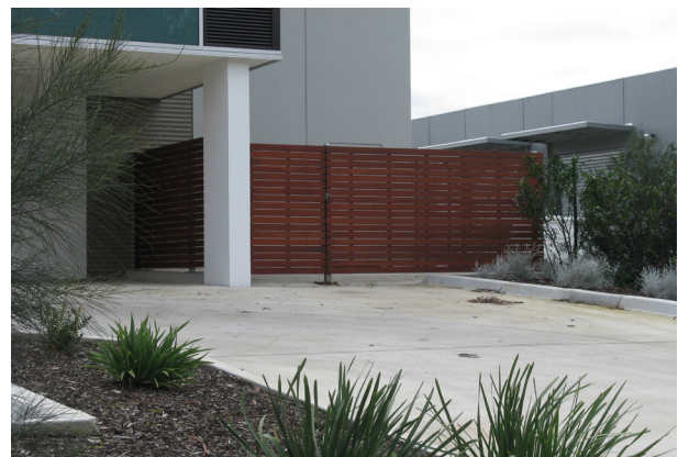
Timber batons provide an aesthetically pleasing screen of a storage area
