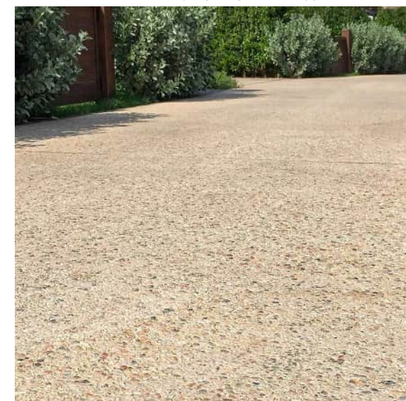
Nepean North & South Exposed aggregate concrete pavement
