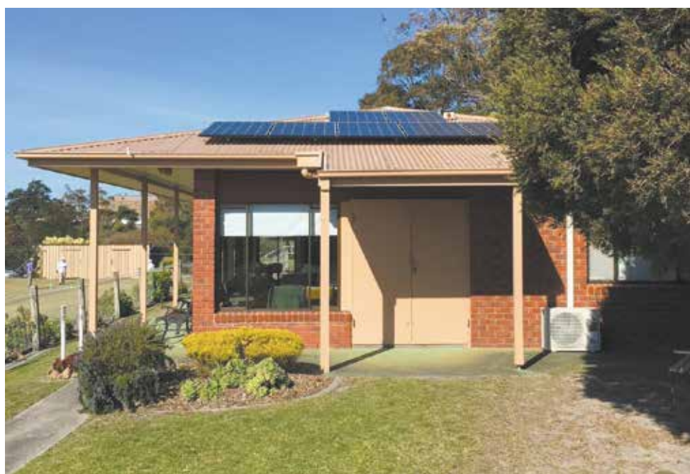
Frankston Croquet Club benefiting from the new solar panels that have been installed.
