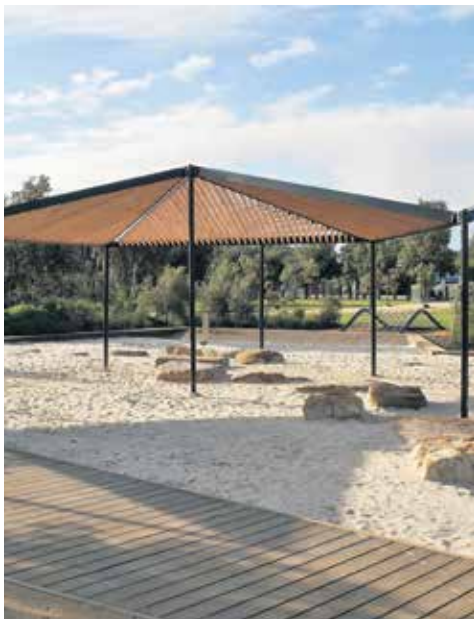
Keast Park shade structure
