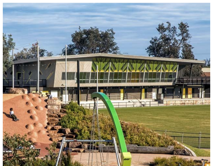
Miles Pavilion is a new 2-storey pavilion with inclusive facilities.
