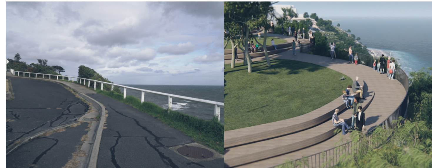
Olivers Hill lookout, before and after
