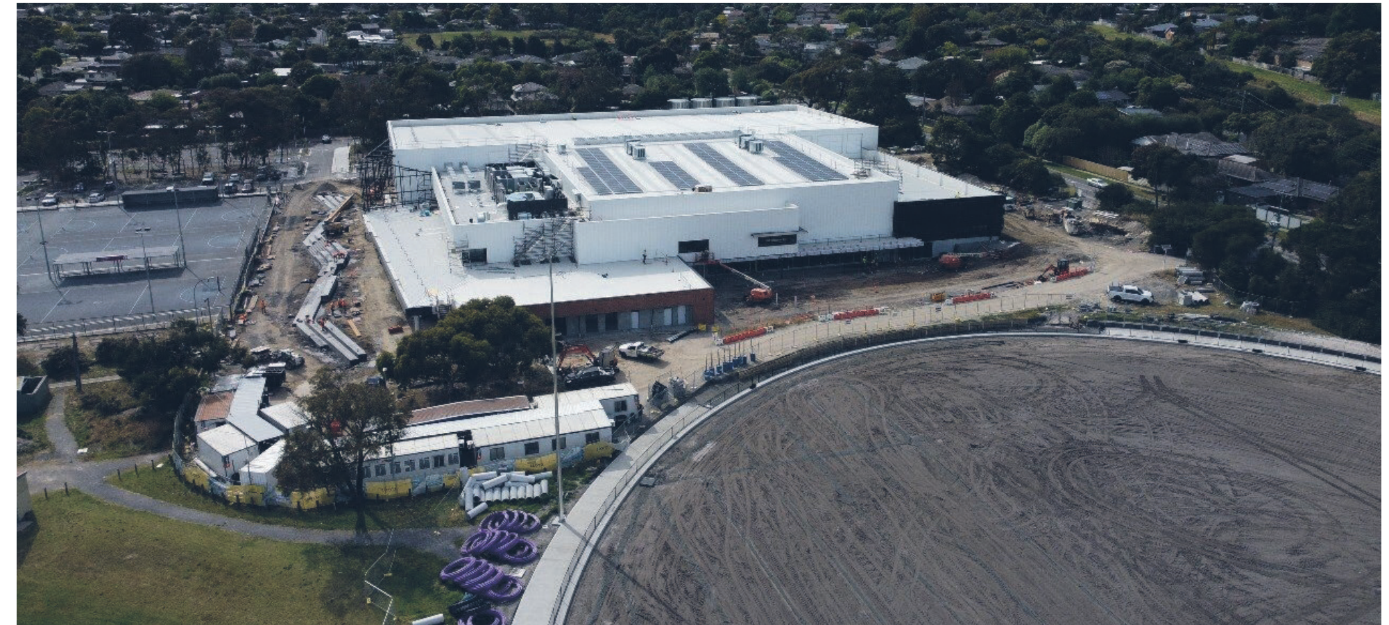
Jubilee Park, captured from above, is nearing completion
