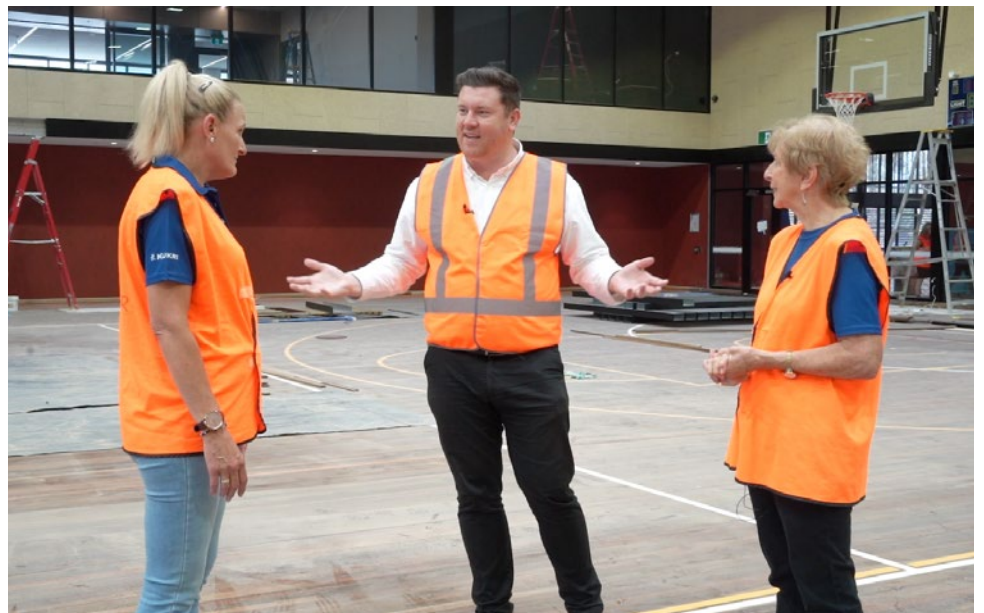
Mayor Conroy visited the Jubilee Park Stadium during construction.
