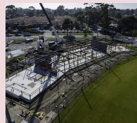
Work has started on the Eric Bell Pavilion.
