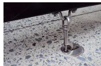
Figure 20: Acceptable Blind Anchor
