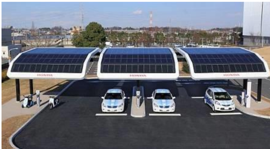
Figure 38: Honda Electric Vehicle Charging Station using solar panels in Europe
