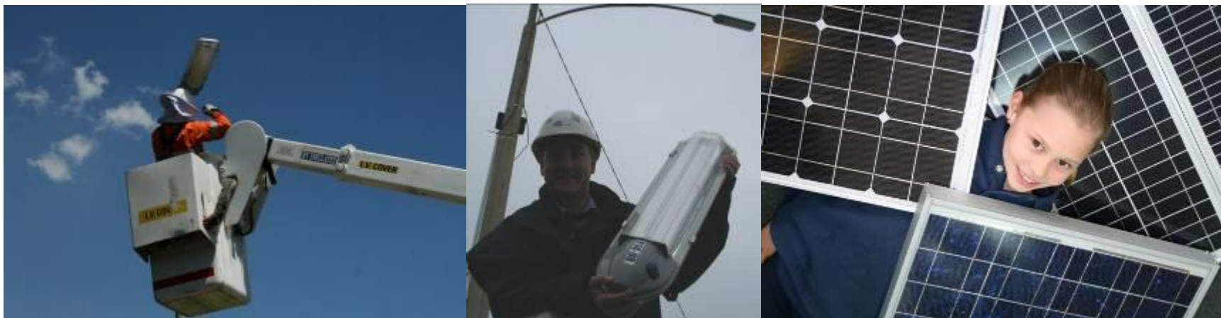
Figure 28: Changing Frankston's streetlights halved energy consumption; community solar programs
