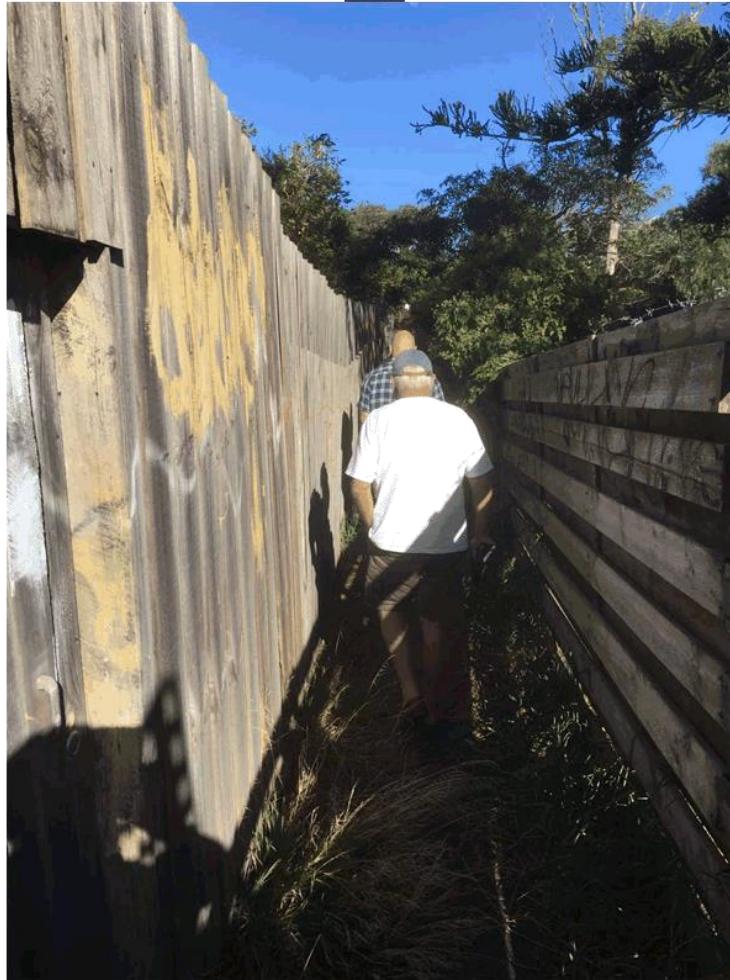
Photo 3 - Highlights the width of the path and the inability to allow pedestrians to pass each other.
