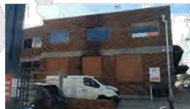
Zone B – Precinct 1: Park Lane
