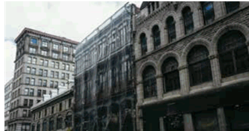
Heritage Building Restoration in Montreal
