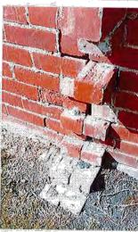
Figure 5: Brick wall bowing
