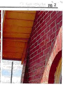
Figure 3: Brick work above arch way level has moved in
