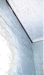
Figure 7: Cracking above arch way at entry, steel plate installed in the past to rectify pervious cracking
