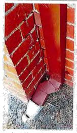
Figure 1: Cracked down pip and separation at corner
