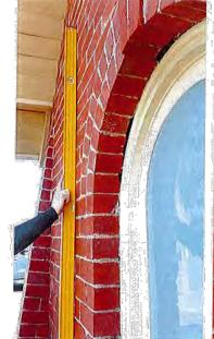
Figure 4: Brick wall bowing
