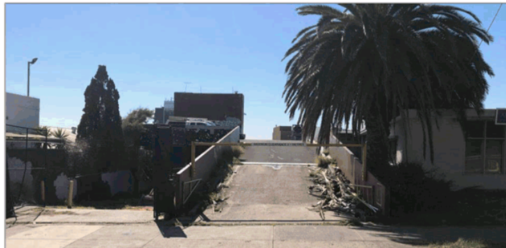
Entry to car park from Davey Street
