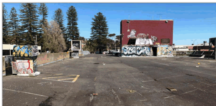
Roof top parking at the site provides for 50 spaces
