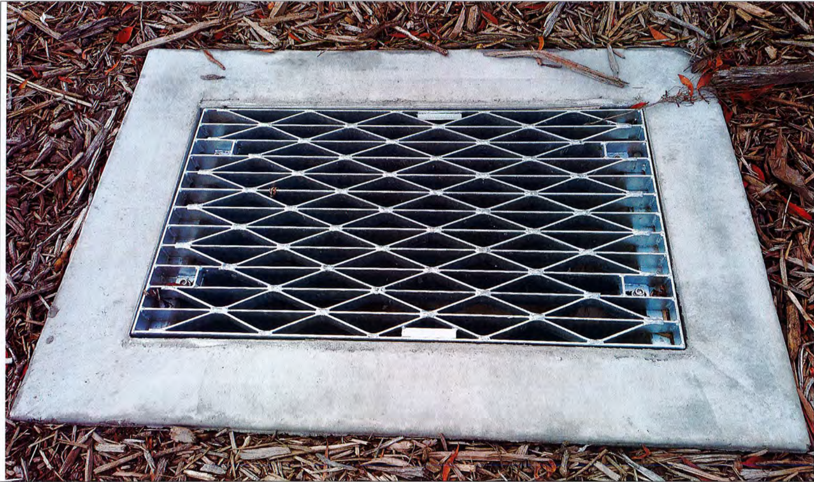
Steel grate with concrete surround
