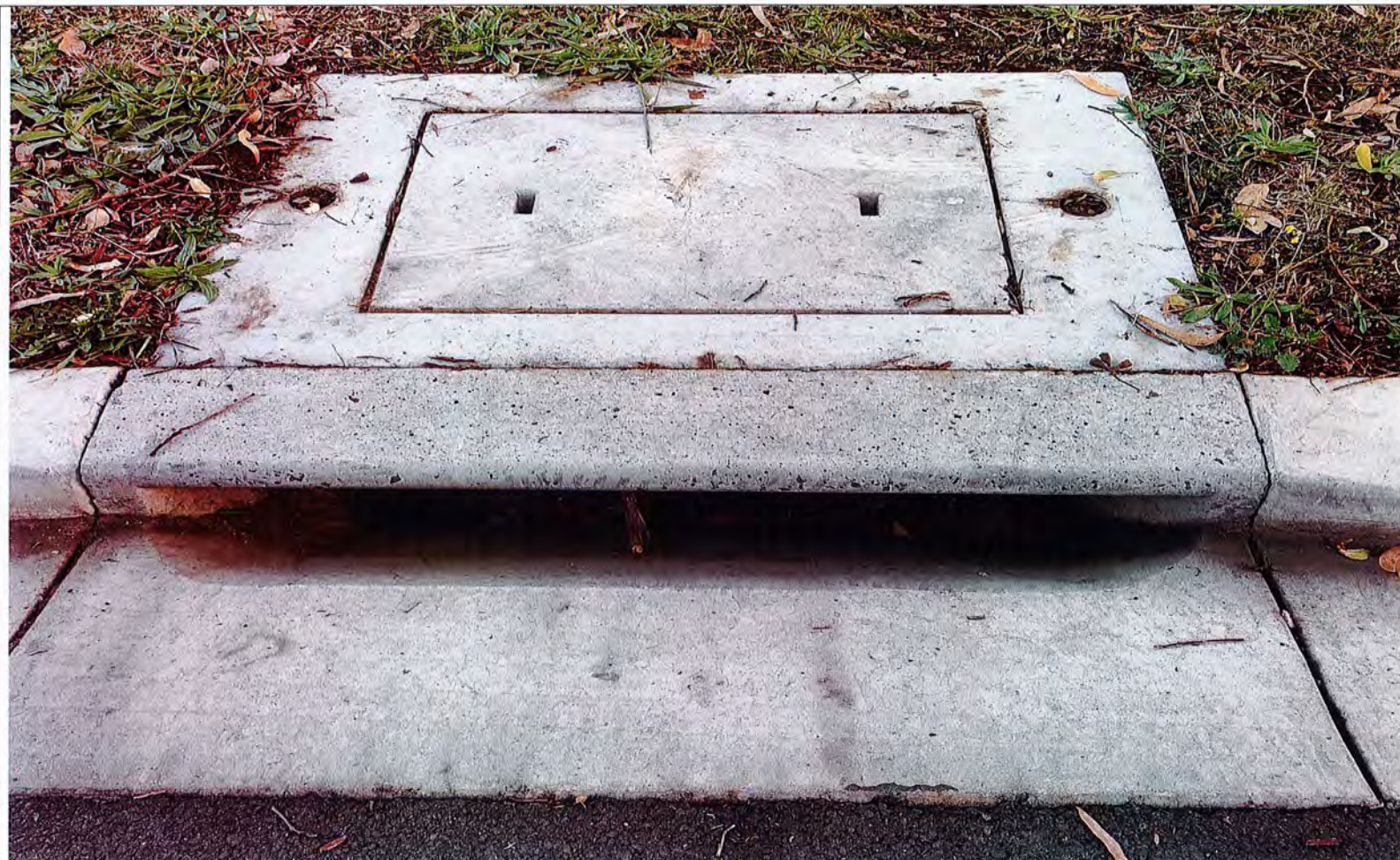
Concrete lintel, surround and access cover
