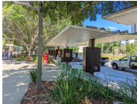
An example of trees, greening and shading to provide a comfortable and attractive transport interchange.
