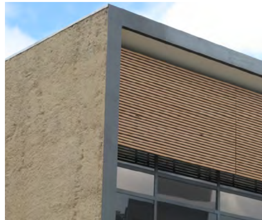
An example of simple detailing and form
