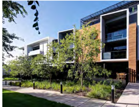
Example of positive street interface with canopy tree planting.
