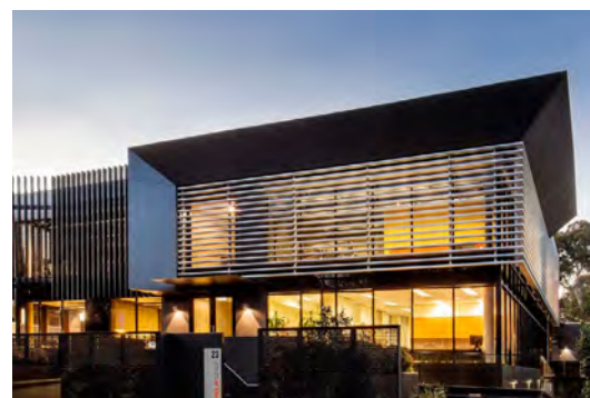
An example of a roof form integrated with the design of the building facade
