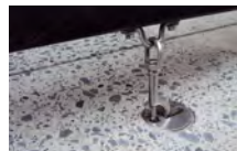
Figure 20: Acceptable Blind Anchor
