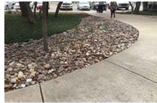
AREAS OF RIVER ROCK PEBBLES OVER UNDERGROUND SERVICES
