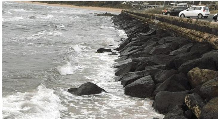
Figure 2.6 Rock deposited in front of seawall
