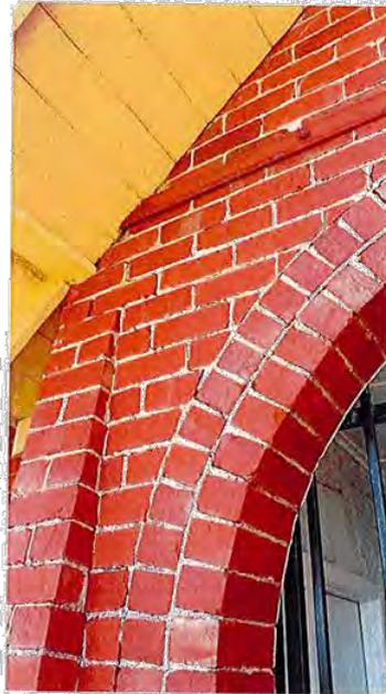
Figure 6: Cracking above arch way, front entry
