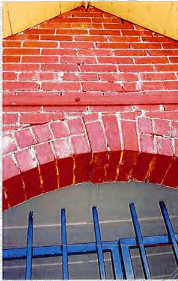
Figure 7: Cracking above arch way at entry, steel plate installed in the past to rectify pervious cracking
