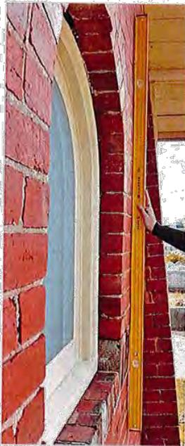
Figure 5: Brick wall bowing
