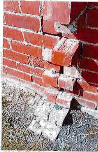
Figure 2: Separation at corner and bricks broken away
