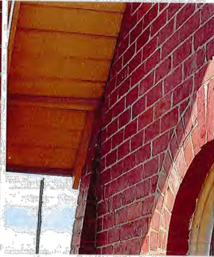
Figure 3: Brick work above arch way level has moved in.
