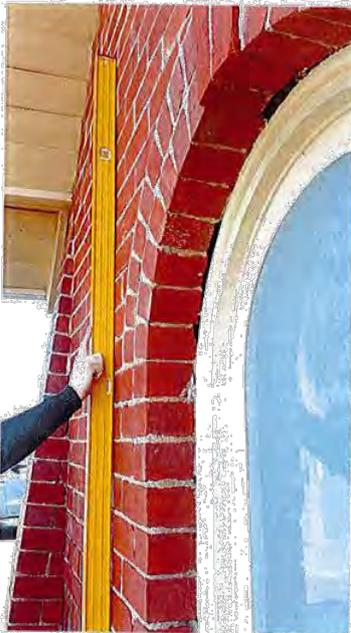
Figure 4: Brick wall bowing
