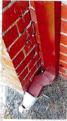
Figure 1: Cracked down pip and separation at corner
